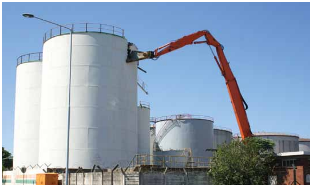
High reach excavator with mechanical shears
