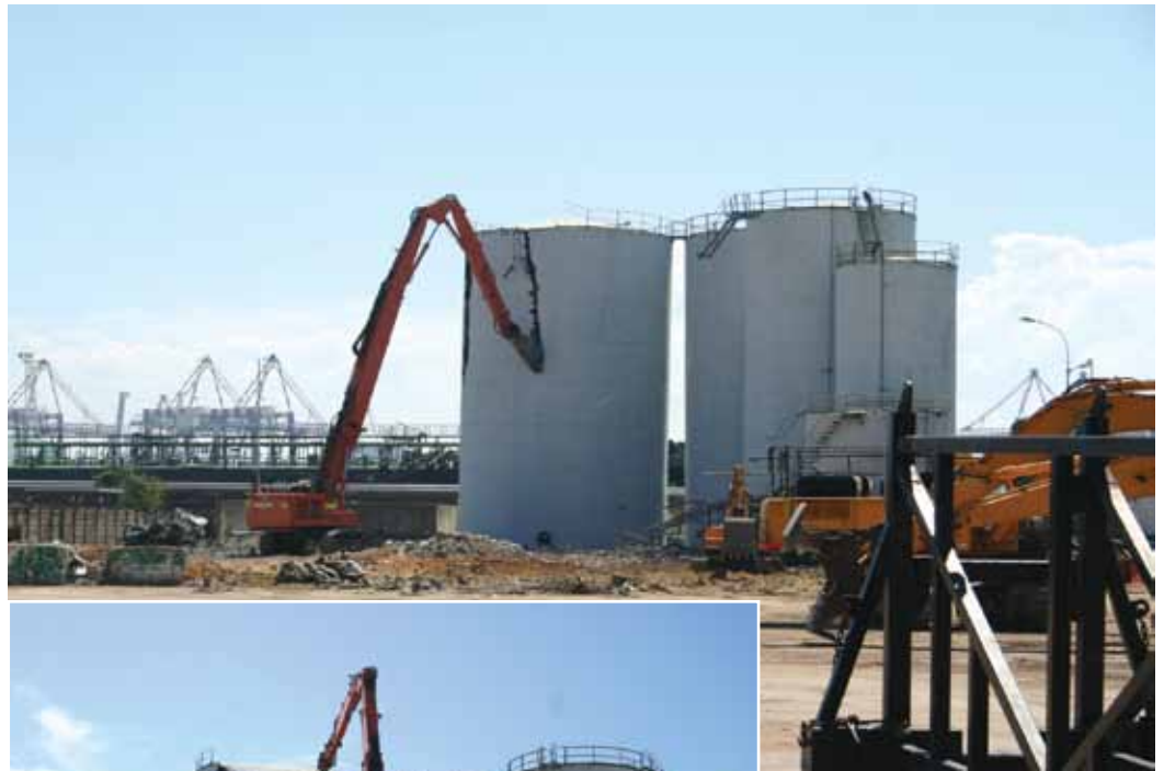
Tank demolition with mechanical shears
