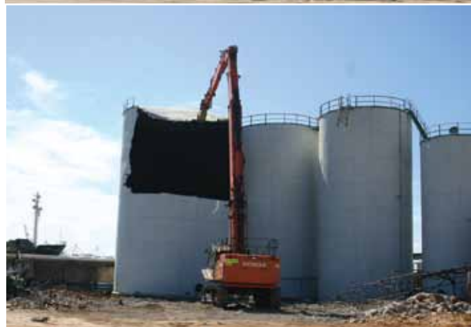
Weaken the tank's structural integrity, then pull the tank on its side
